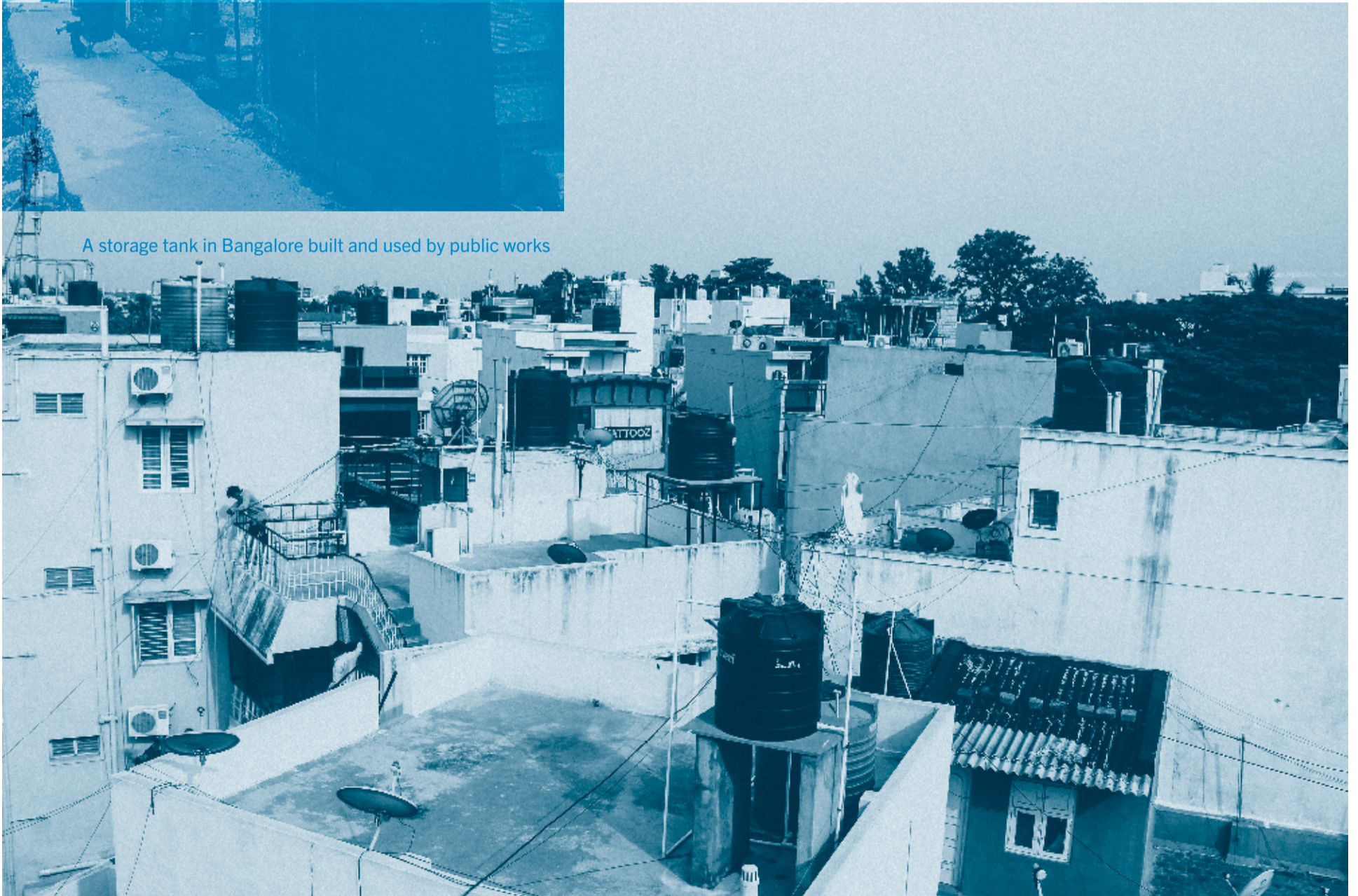
Overhead water tanks in a Bangalore neighbourhood
