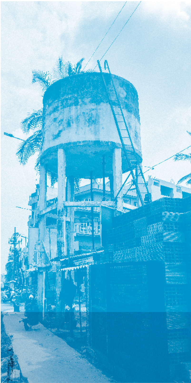
A storage tank in Bangalore built and used by public works
